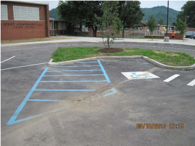
Picture – 13: Photo of ADA parking space & loading zone at parent drop-off loop lacking signage and with low area.
