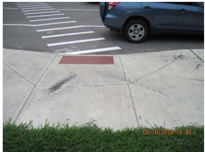
Picture – 24: Photo of cracked sidewalk @ ADA ramp.
