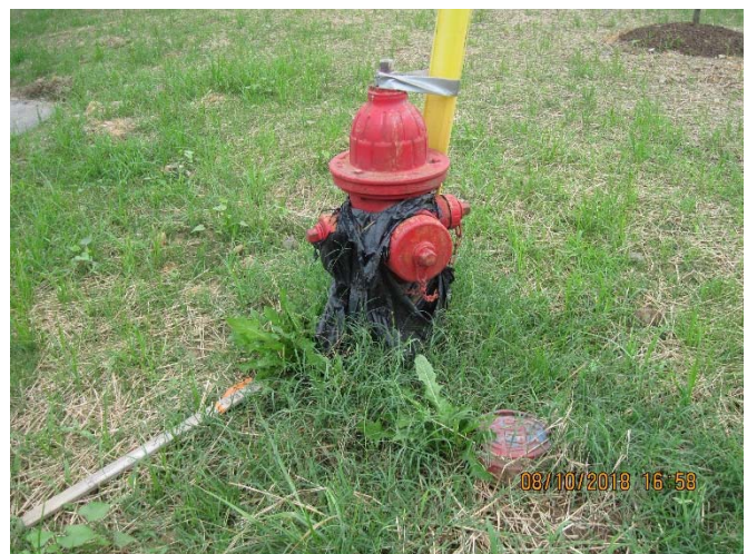
Picture – 30: Photo of fire hydrant which protection can be removed and hydrant cleaned..
