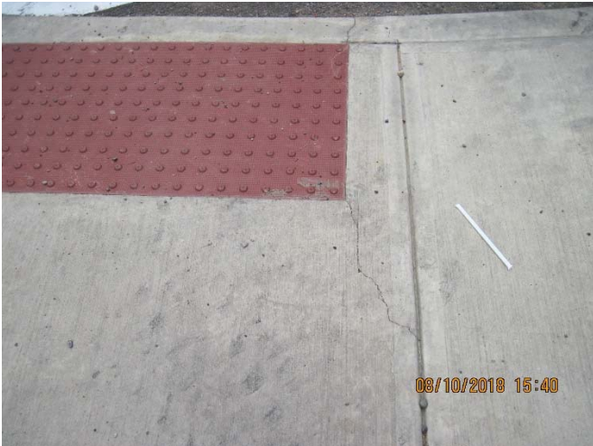
Picture – 25: Photo of cracked sidewalk @ ADA ramp.
