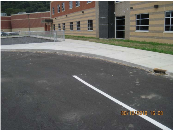
Picture – 15: Photo of uneven curb height and of abrupt high spot in concrete sidewalk.
