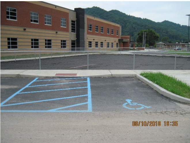
Picture – 12: Photo of ADA parking & loading zone without signage & very dirty pavement.
