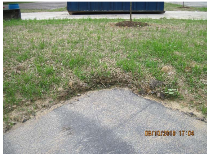
Picture – 29: Photo of corner of parking space where grade is too abrupt at corner and soil should be excavated & removed.
