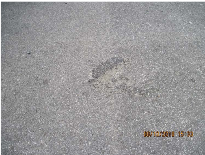
Picture – 20: Photo of scrape / divot in new pavement.
