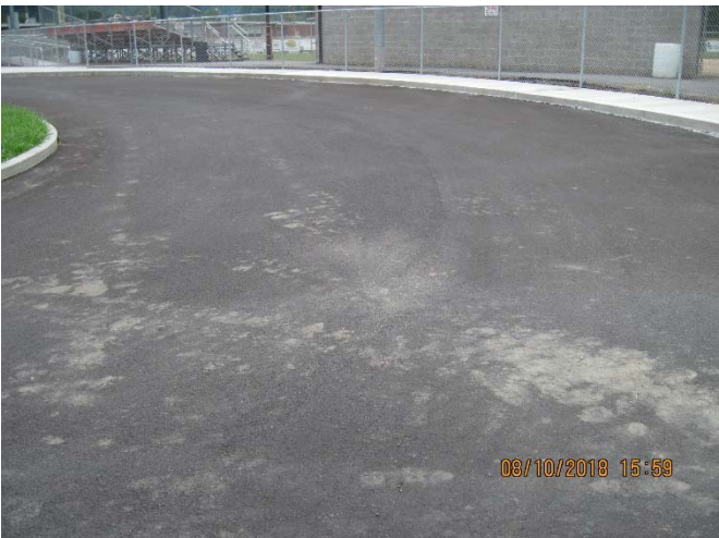
Picture – 18: Photo of low spot & dirty new pavement.
