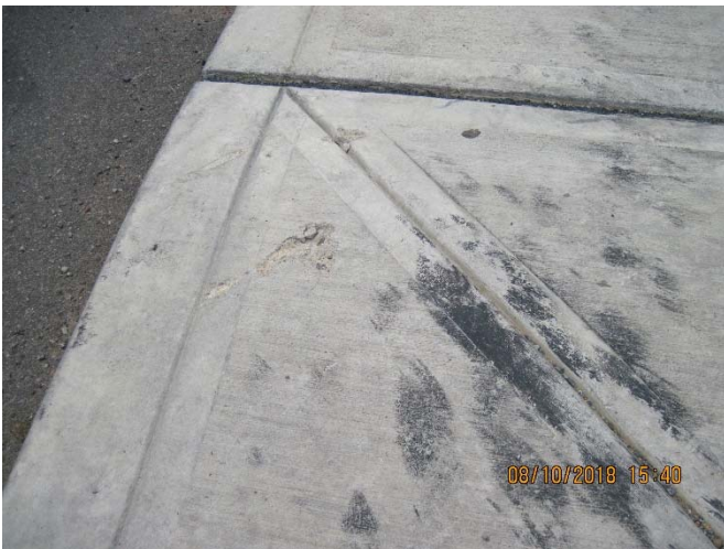
Picture – 26: Photo of chipped concrete sidewalk @ ADA ramp.
