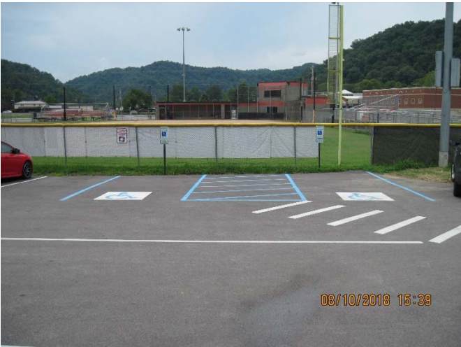
Picture – 11: Photo of ADA parking spots across from elementary school which lack a sign at the loading zone.
