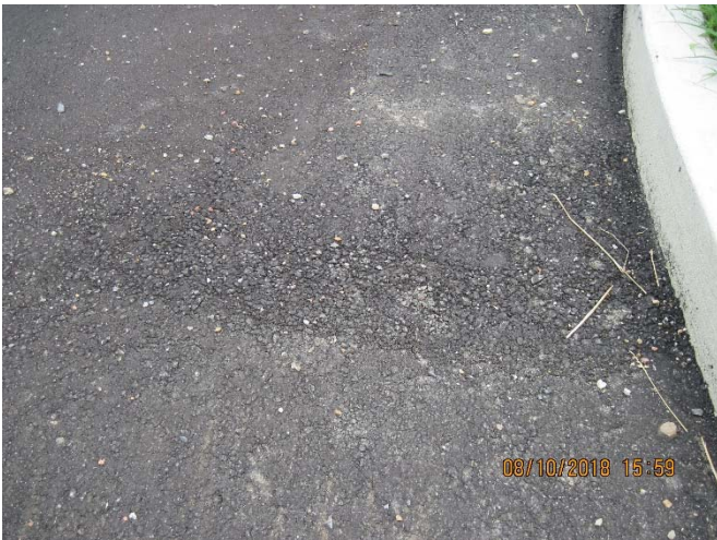
Picture – 14: Photo of rough wearing course pavement found at bus loop.
