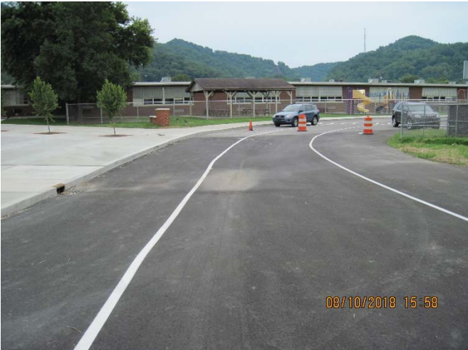
Picture – 16: Photo of low spot in pavement.
