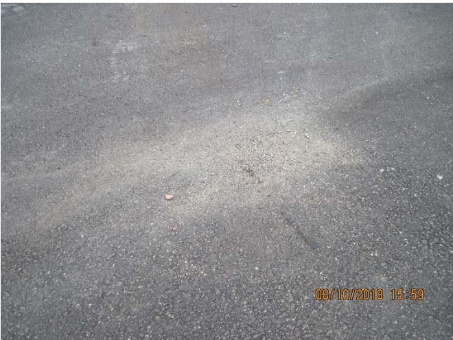
Picture – 17: Photo of low spot in pavement.
