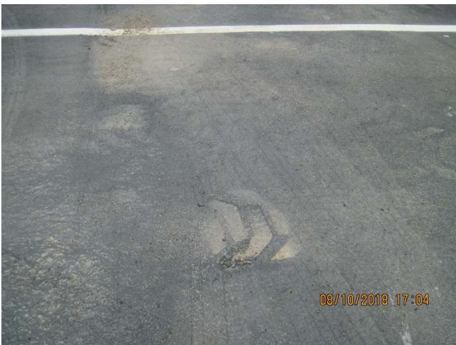
Picture – 21: Photo of tire imprint & low spot in pavement.
