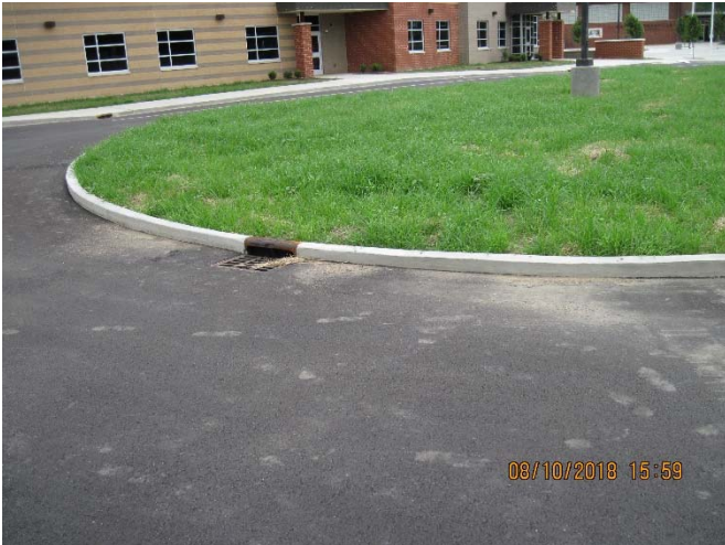
Picture – 19: Photo of low spots along curbing to CB A7..
