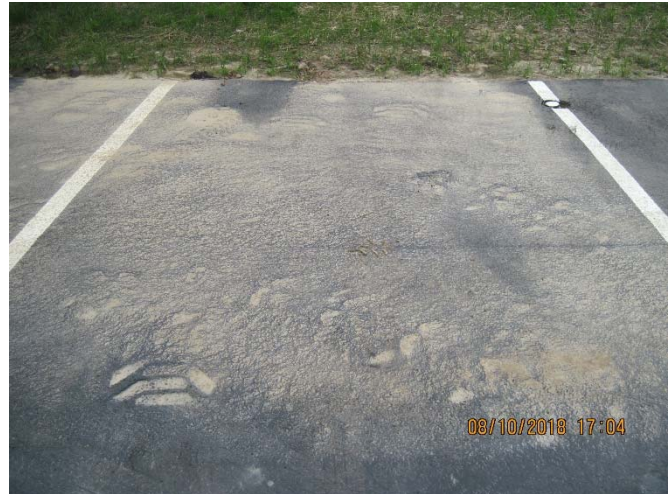
Picture – 22: Photo of tire imprints & divots in new pavement.
