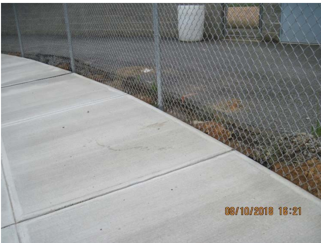
Picture – 27: Photo of gap between sidewalk & fencing which should be filled.
